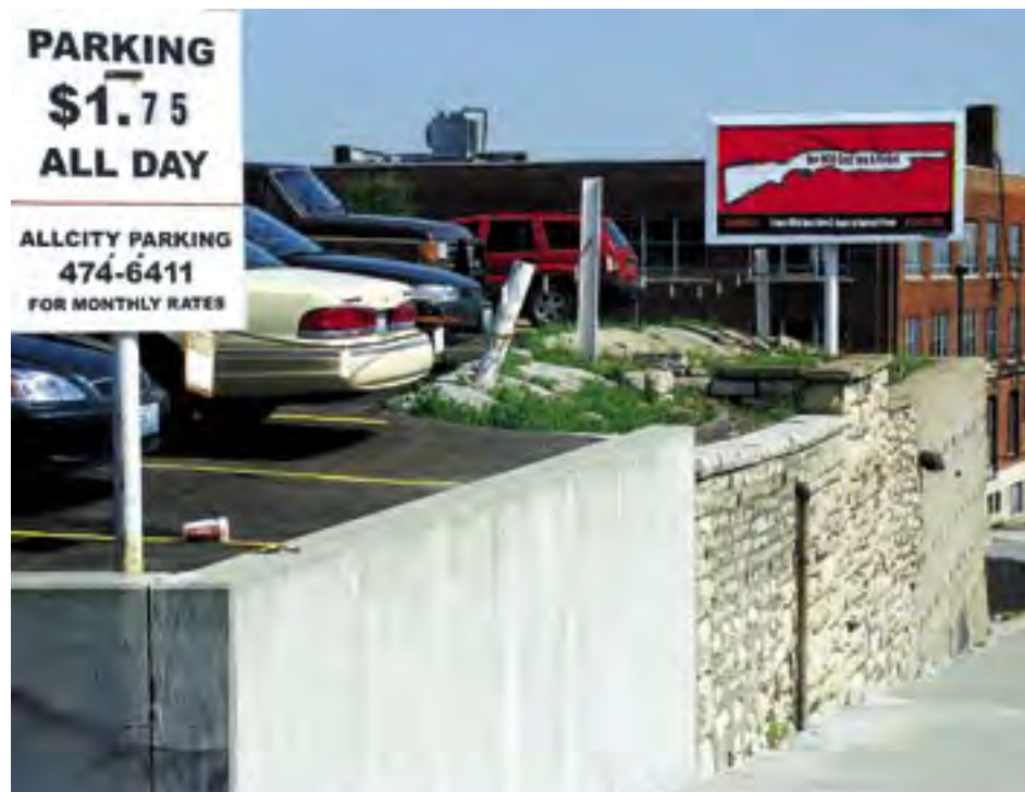
Retaining walls and building foundations around Mcgee, between Admiral and 8th St. (Photo: James Woodfill)
